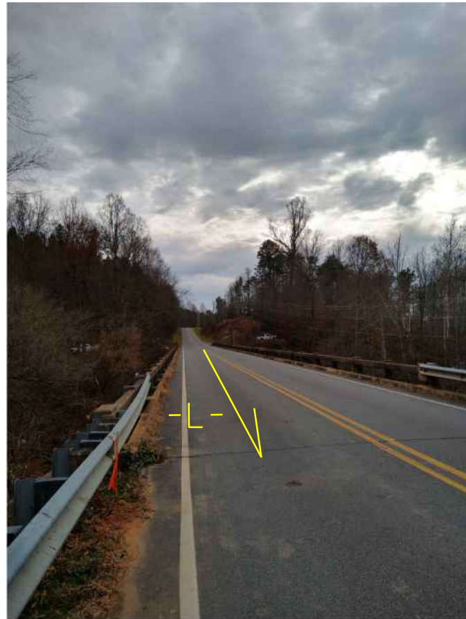
Photo #1: End Bent 2 looking south (downstation)
