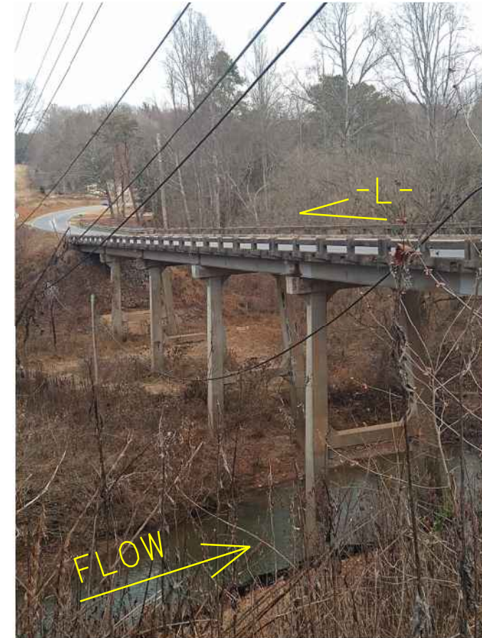
Photo #2: End Bent 1 looking north/northeast (upstation)
