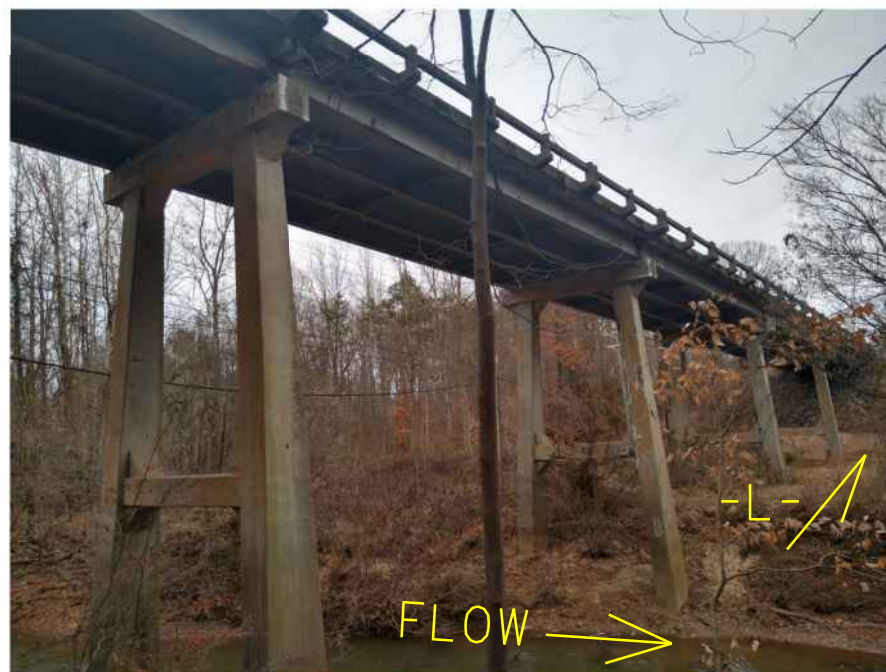
Photo #3: Right side of existing bridge looking north/northwest (upstation)
